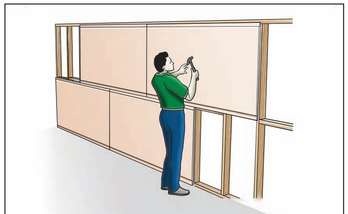
FIGURE 5 FIXING REMAINING SHEETS
